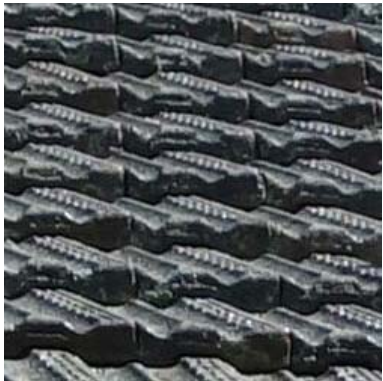
1. EXISTING ROOF TILES
