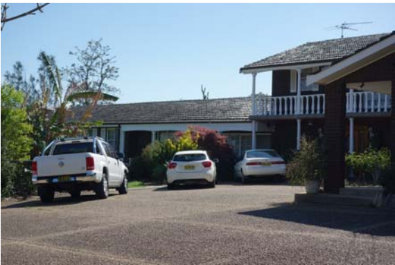
VIEW C - FRONT FACADE, EXISTING
