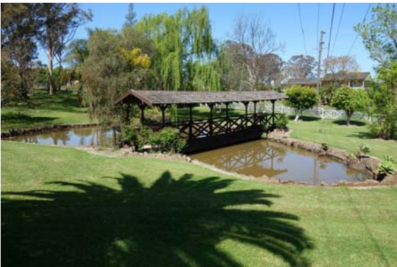
VIEW D - EXISTING POND
