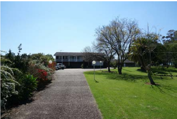
VIEW B - EXISTING DRIVEWAY
