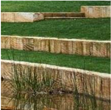
11. SANDSTONE RETAINING BLOCKS
